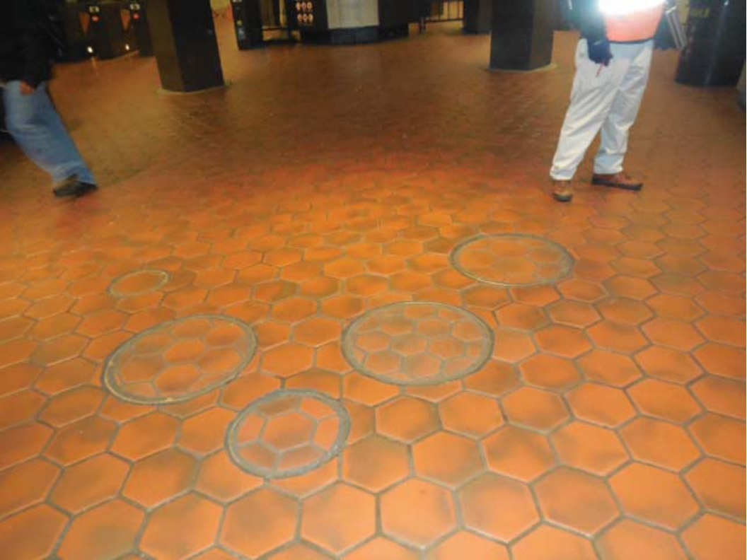
Picture 1: C05 Rosslyn – Handholes in mezzanine on paid side
