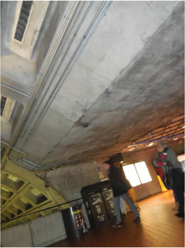
Pictures 5-7: C04 Foggy Bottom – Conduits on Mezzanine ceiling and passing through drop ceiling
