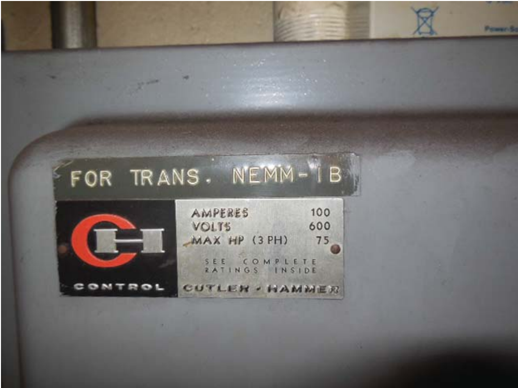
Picture 10: C02 McPherson Sq (East) – Disconnect switch for Trans NEMM-IB in room 211
