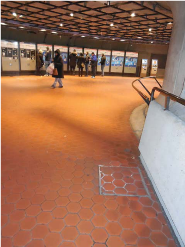
Pictures 1&2: C04 Foggy Bottom – Handholes in Mezzanine
