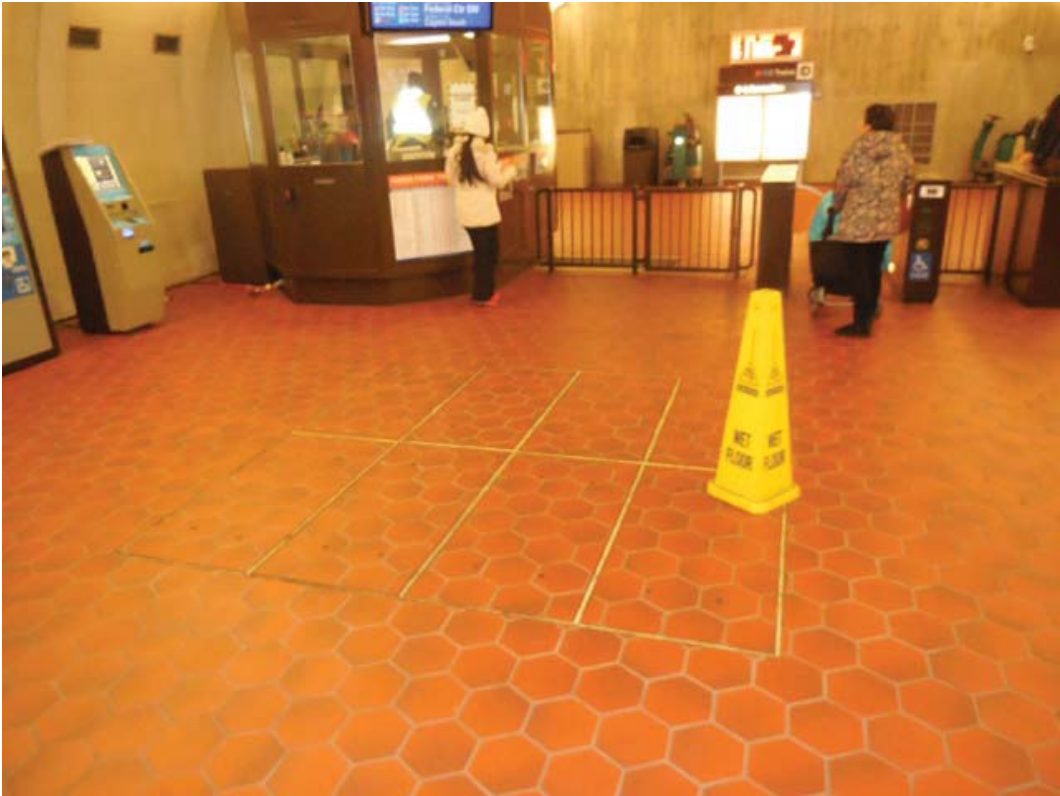
Pictures 1&2: C05 Rosslyn (NEW) – Handholes in mezzanine
