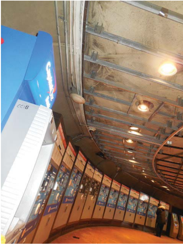
Pictures 5-7: C04 Foggy Bottom – Conduits on Mezzanine ceiling and passing through drop ceiling
