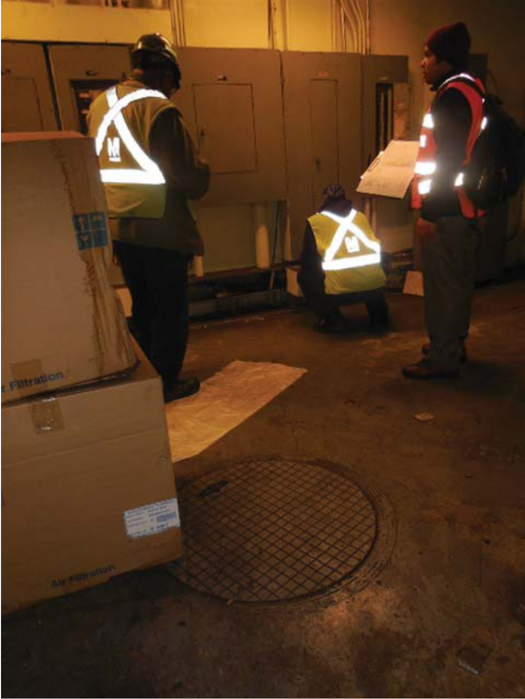
Picture 10: C04 Foggy Bottom – Manhole in room C204
