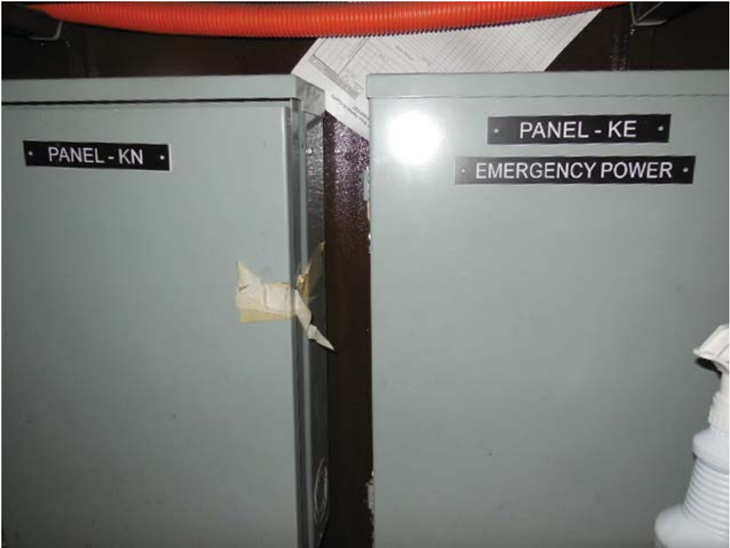
Picture 4: C05 Rosslyn (NEW) – Emergency Panel KN and Panel KE in Kiosk
