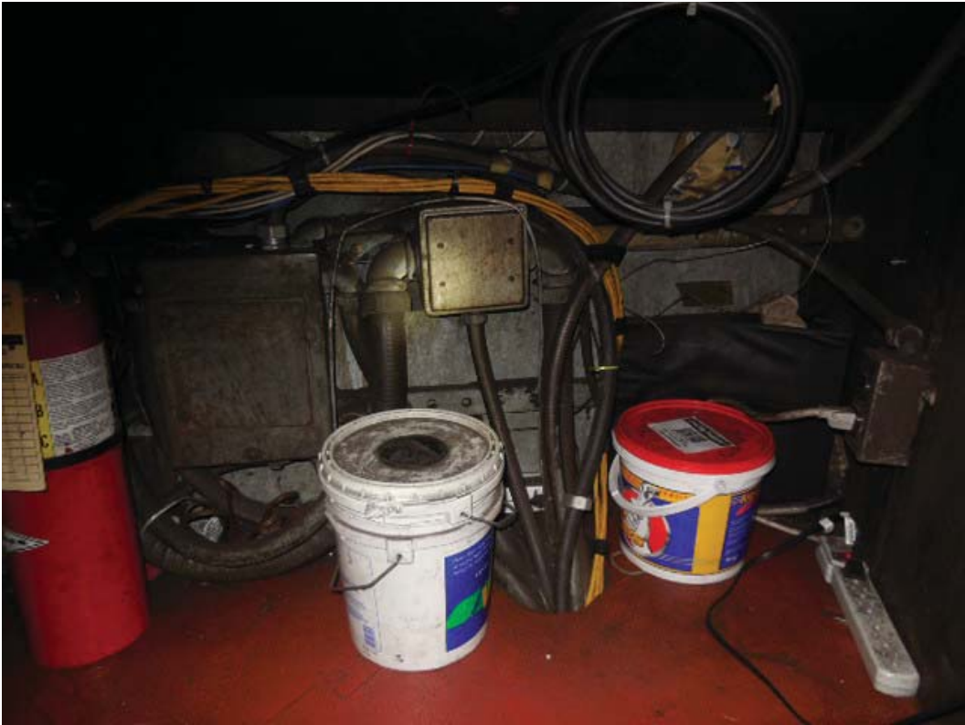
Pictures 3&4: C03 Farragut West – Emergency panel in Kiosk
