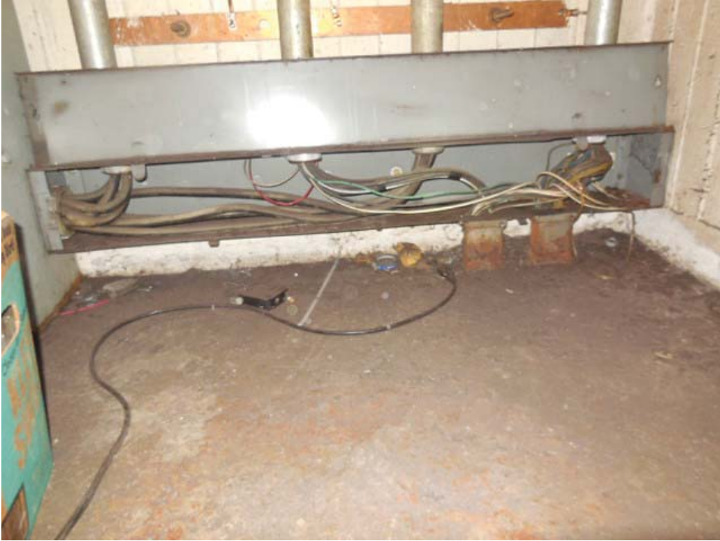
Pictures 8&9: C05 Rosslyn – Shared trough for panels F1 & F2 in room C304
