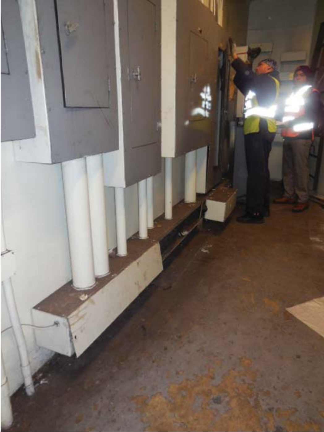
Picture 22: C04 Foggy Bottom – Common trough for multiple panels in room C204
